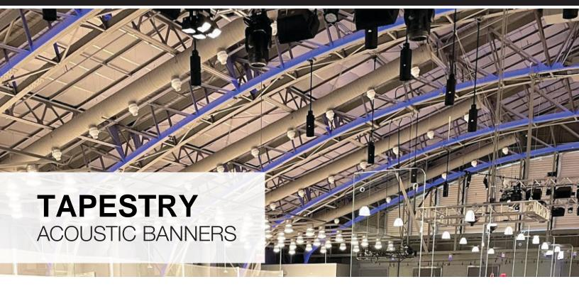
NetWell Tapestry Banners are the perfect economical solution to reverberation issues for large spaces. They are easy to install horizontally with the ceiling via grommets or aluminum stiffener bars. Spacing the distance of the fixed ends will control the droop height. The Tapestry Banners are custom made with a wide variety of finishes and sizes available.
